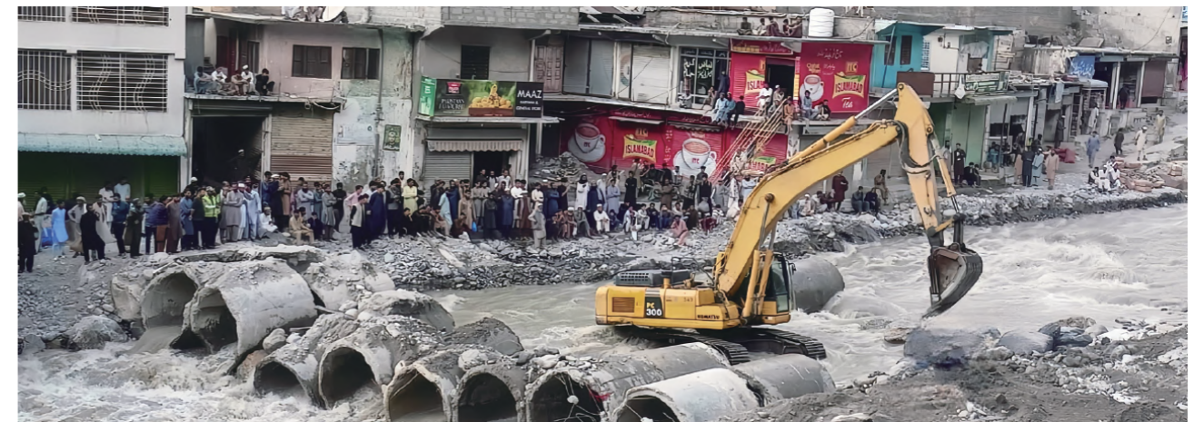
Figure: SK Project Repairing Bridges in the Mahandri Area
