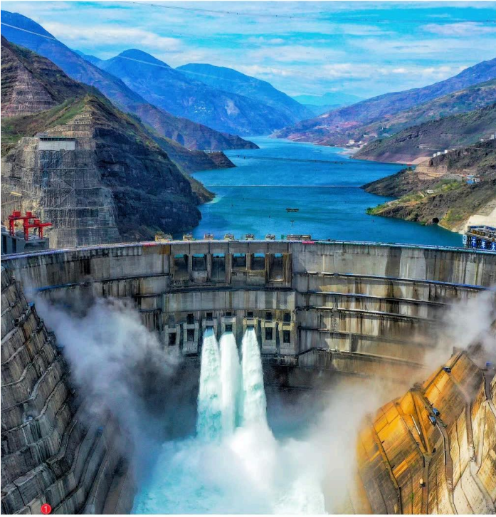
Baihetan Hydropower Station in China (Participation in construction)
