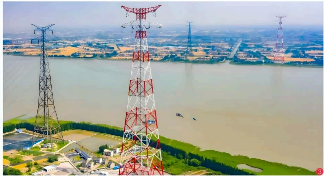
Fengcheng - Meili 500kV Yangtze River Crossing Project in China (Design) 中国凤城 - 梅里 500kV 长江大跨越工程 (设计) 3. With an operating voltage of 500kV, the Project is the largest UHV transmission and transformation project crossing the Yangtze River in China. 500kV，中国规模最大超高压跨越长江输变电工程。
