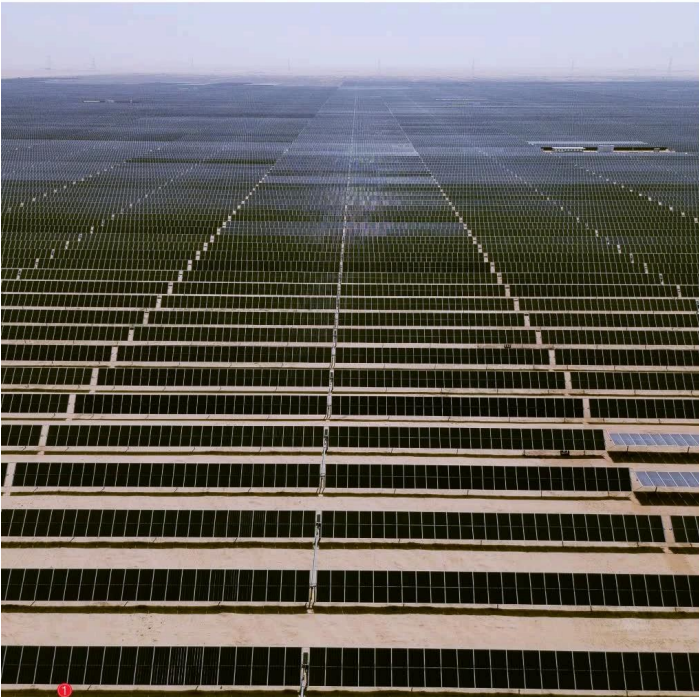
1 Al Shuaibah 2.6GW Photovoltaic Power Plant Project in Saudi Arabia (EPC) 沙特阿舒巴赫 2.6GW 光伏电站项目 (工程总承包) With an installed capacity of 2.6GW, it represents the largest PV project in the Middle East. 2.6GW, 中东最大光伏项目。
