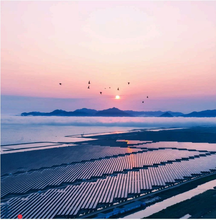
1 500MW Fishery-PV Complementary Power Generation Project in Haiyan Town, Taishan City, Guangdong Province, China (Participation in Investment and Construction) 中国广东台山海宴镇 500MW 渔业光伏发电项目 (参与投资建设) With an installed capacity of 500MW, it is the largest single contiguous fishery-PV complementary integration project in Guangdong-Hong Kong-Macao Greater Bay Area. 500MW, 中国粤港澳大湾区单体连片规模最大渔光互补一体化项目。
