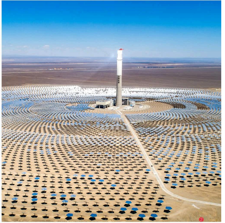
2 50MW Molten Salt Tower CSP Power Generation Project in Hami, Xinjiang, China (Investment and Construction) 中国新疆哈密熔盐塔式 50MW 光热发电项目 (投资建设) With an installed capacity of 50MW, it is among inaugural batch of 20 CSP demonstration projects in China. 50MW, 中国首批 20 个光热示范项目之一。
