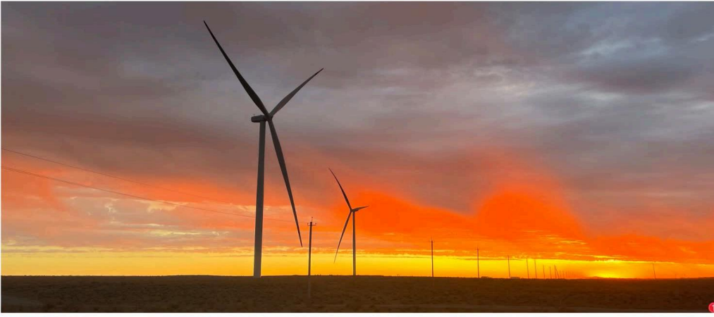
Bukhara IGW Wind Power Project in Uzbekistan (EPC) 乌兹别克斯坦布哈拉 1GW 风电项目 (工程总承包) ① With an installed capacity of 1GW, it is the largest wind power project currently under construction in Central Asia. 1GW, 中亚在建最大风电项目。
